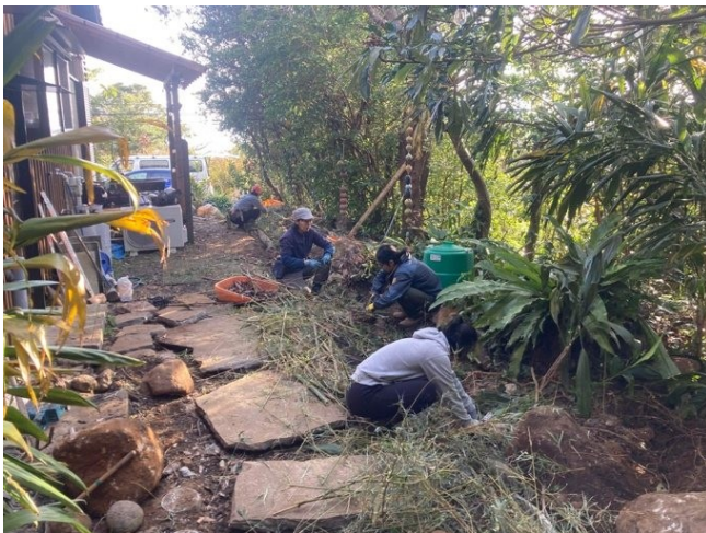
Breaking a once-solid path to let air and water flow. Photo: Wakuworks
