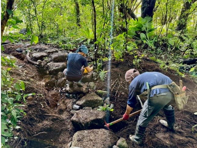
Building a path to the Commons. Photo: Wakuworks
