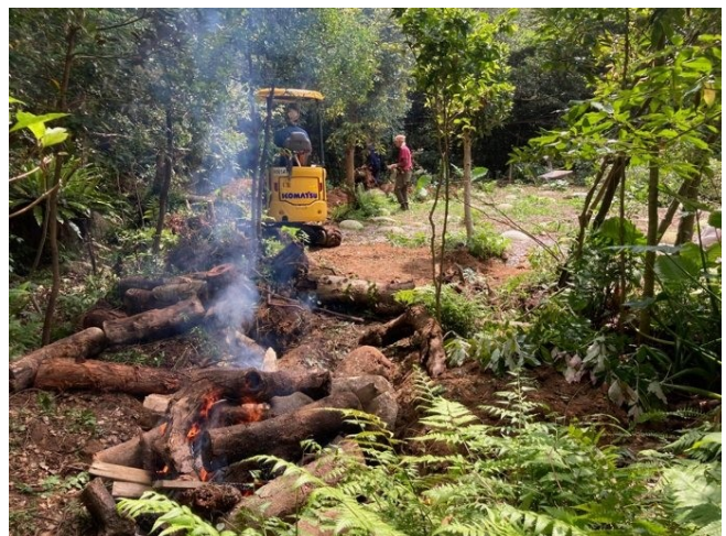
Making charcoal for the air-and-water veins. Photo: Wakuworks
