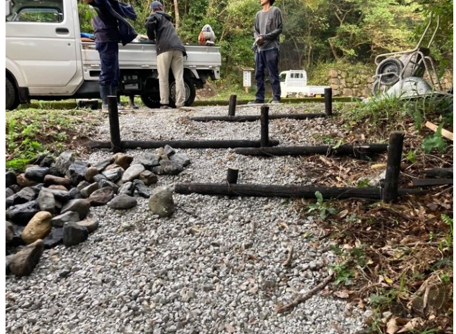
Building the stone road from Route 77 to the Commons and Crossroads. Photo: Wakuworks
